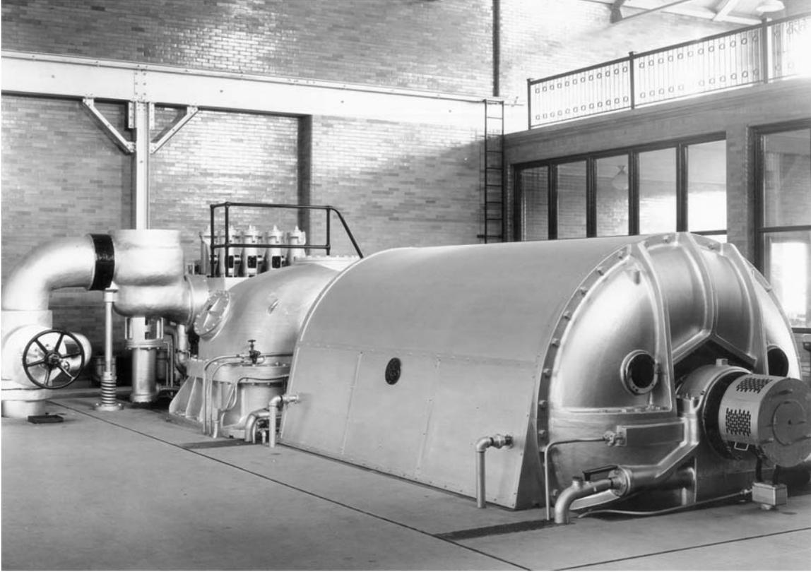
The 15,000 kw machine was carrying the entire load of the city. In reserve were the 10,000 kw machine and the 5,000 kw turbo generator, both of which were rebuilt during the improvement program.
